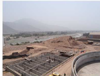
Santa Clara WWTP (in construction) ifak
