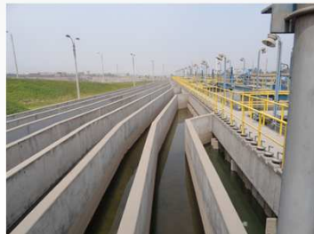
Huachipa WTP (in construction)
