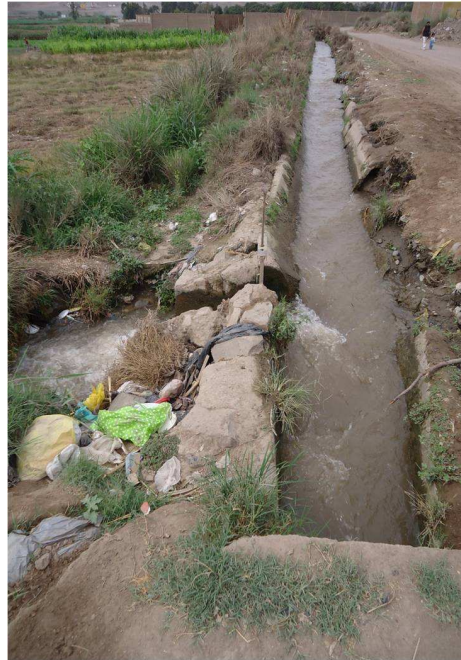
Figure 2.8: The network of canals which passes through Chuquitanta carries water diverted from the Chillón River for use in flood irrigation of local agriculture; the opening and closing of sluice gates along the network controls the inundation of field parcels. [57] [photo: ILPÖ]
