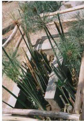
(a) Concrete basin with plantings as constructed wetland “module” [photo: [107]]
